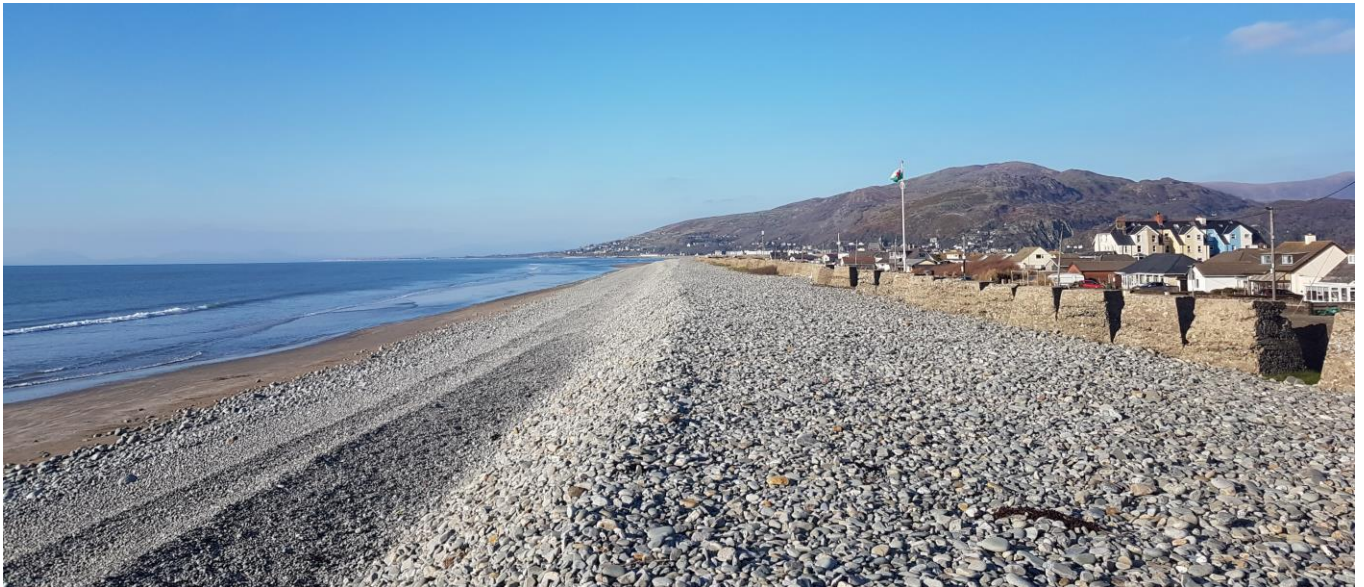
Figure 3. The shingle bank that defends Fairbourne consists out of shingles (rounded pebbles) that have eroded from nearby cliffs and have collected onto the beach due to the waves. On the left of the shingle bank is the beach, which is submerged during high tide. Houses in the village Fairbourne can be seen on the right of the shingle bank. On top of the shingle bank are “dragon’s teeth”, remaining as war defences from the Second World War (taken on March 2, 2023).
